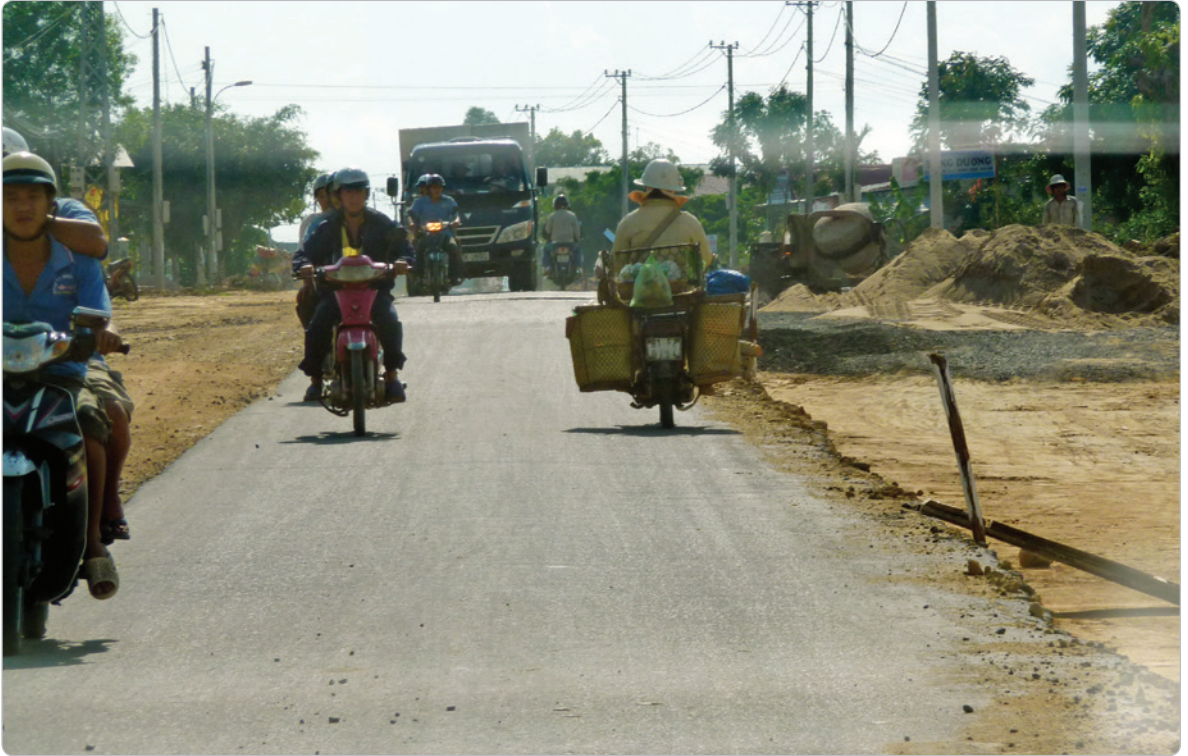
Besides the new power house the project has also funded the construction of roads, bridges, canals and even a school in the local communities.
